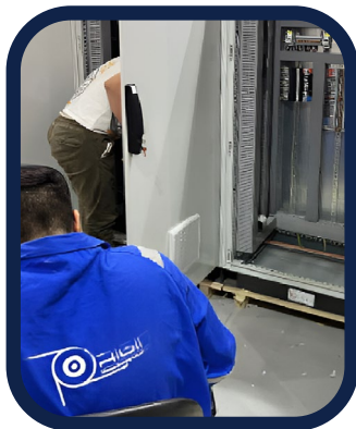
APS Material installation
